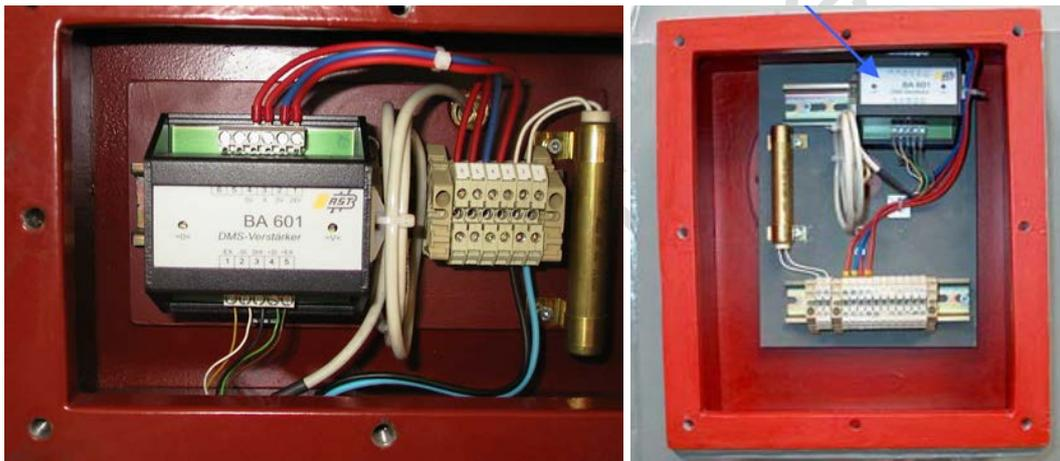
Figure 1: Installation examples for BA 601
