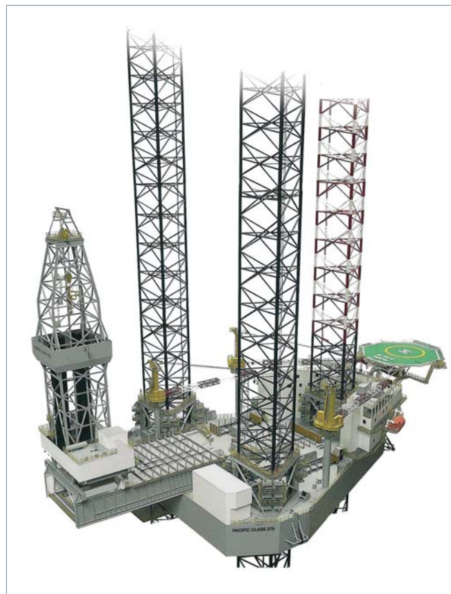
Above: BMC Pacific 375 deep drilling offshore jack-up rig designed and delivered by PPL shipyard, Singapore
